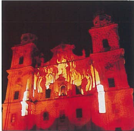
Donnellan's earlier project in Salzburg Cathedral Square where Pani projectors were used to light the facade.
